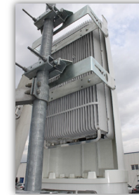
Nokia radio into the Hybrid Kit
